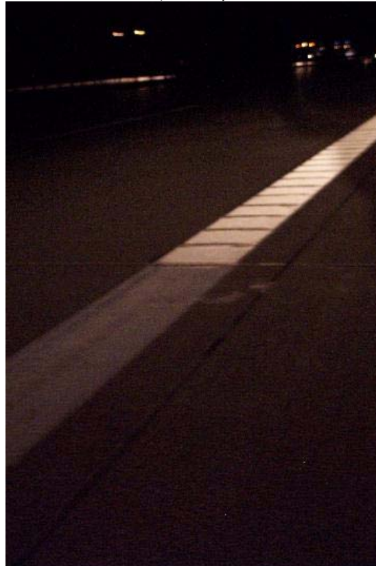
Cross point border marking Paint/ CP 90°cross-profiled on freeway A 2 at night, direction Hannover, km 15,3
