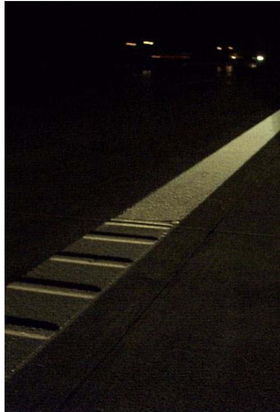
Cross point border marking CP profiled/ CP Agglomerate on freeway A 2 at night, direction Hannover, km 5,0
