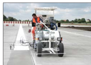
H26 in Saint Petersburg/Russia equipped with 1-component cold paints as well as sprayable 2-component cold plastics Airless system 98:2, 460 lts pressurised container, for use with one paint gun resp. 2-component spray gun for taxiways
